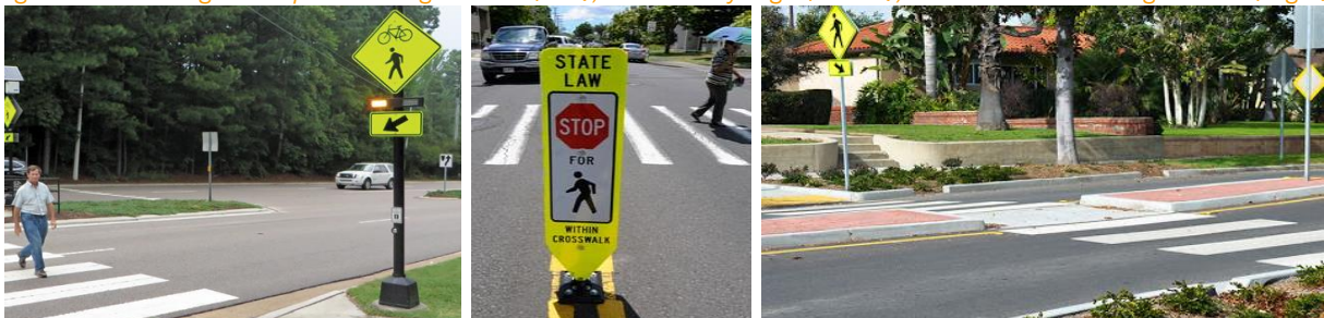
Figure 90: Rectangular Rapid Flashing Beacon (Left), In-Roadway Sign (Center), and Pedestrian Refuge Island (Right)
