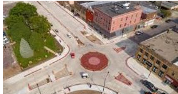
Figure 86: Mini Roundabout in Downtown St. James, MN
