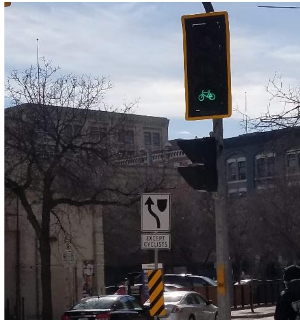
Figure 112: Bicycle Signals in Winnipeg, MB
